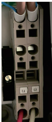
Figure 4.10 AC Connection Area of Inverter
